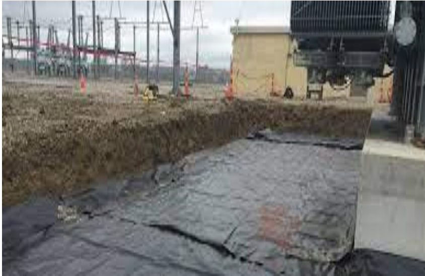
FIGURE 8 Secondary Containment Coatings & Repair Work Solution (Google image, 2020)
